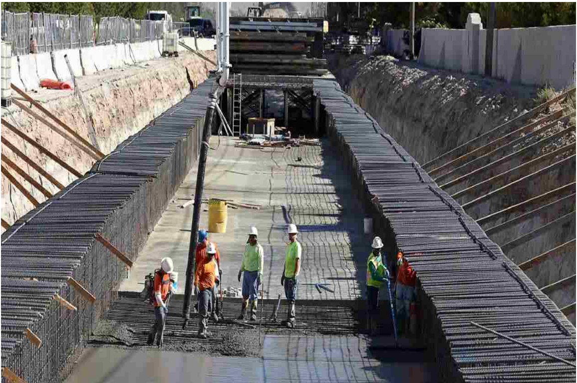
Figure 11. Workers building an underground storm drain in Northwest Las Vegas. (image courtesy of CCRFCD)
