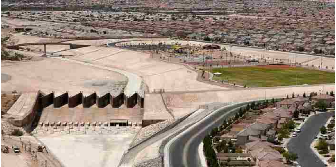
Figure 8. Lower Las Vegas Wash Detention Basin (image courtesy of CCRFCD)
